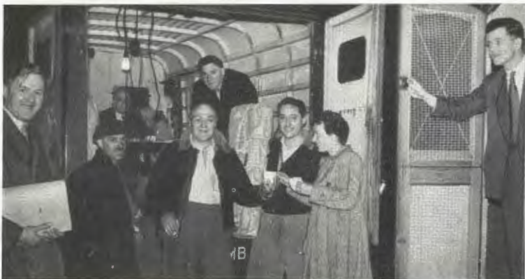
Our photograph shows electricians Messrs. Ashurst and Waller collecting materials for the next job including a "cup of char" which chargehand Hutchinson passes to them from Miss Scott (lady demonstrator). Foreman Mr. Atkinson in the background is making out the documentation while Driver J. Wells assists with sorting out the fittings. Mr. D. E. Jones, Service Centre Supervisor (right), is eagerly awaiting the next orders being brought in by Mr. Kirkham (Warrington Service Centre).
