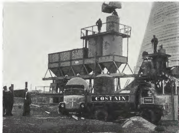
Mixing the concrete at Bold Power station, where extensive use of P.F.A. was made.
