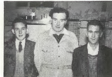
Contracting Department staff from Lister Drive who were responsible for installation arrangements at the Prescot exhibition. Left to right Messrs. E. R. Bostock, G. H. Jones and P. Brogan.
